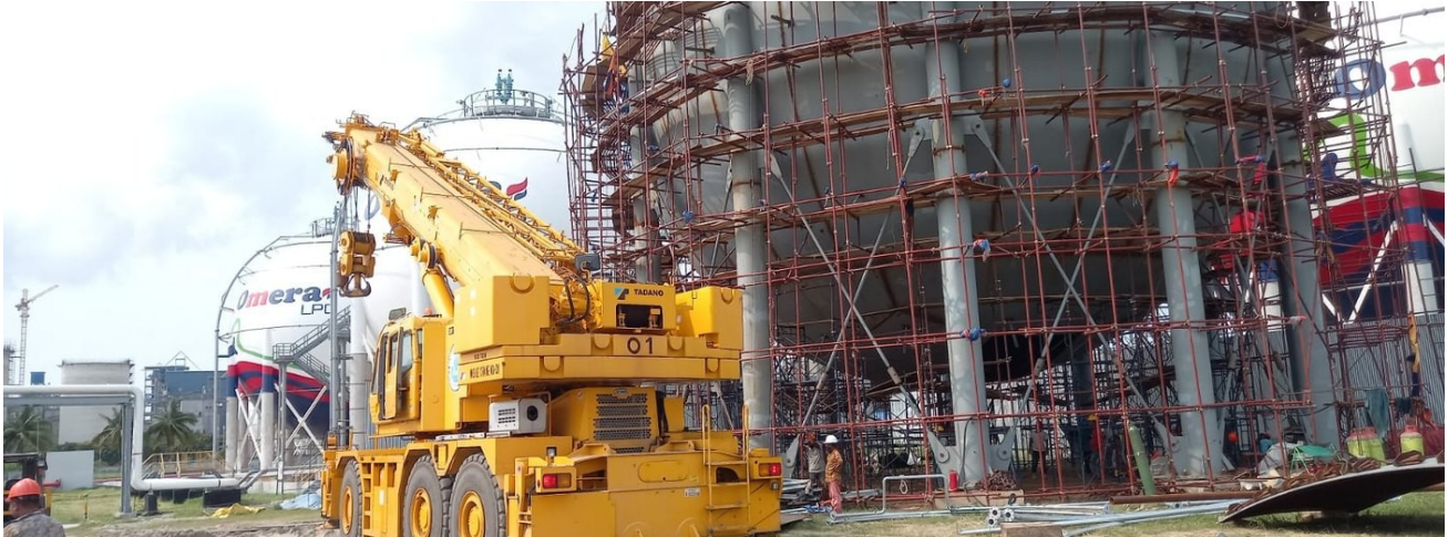
01 Crane support at a spherical tank construction site
