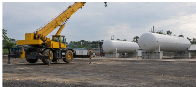
03 Crane support for bullet tank installation
