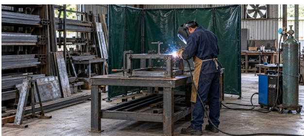
06 Steel fabrication and welding
